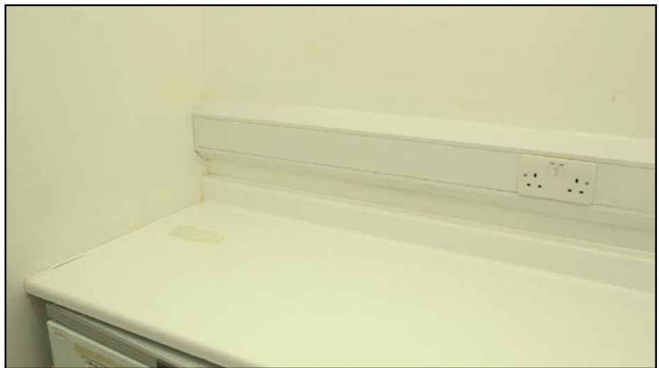
Figure 8 Bench surface sealed to wall
